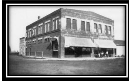
Hoskins and DeSart building (now the Center Market)
